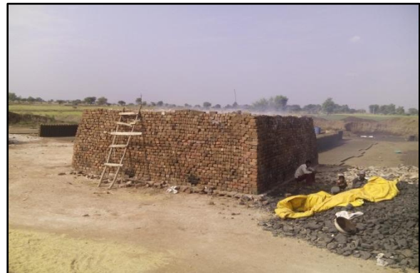
Fig. 4 Kiln for baking bricks
